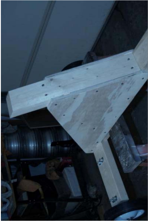
Seat Post and Brace – Both side panels installed
