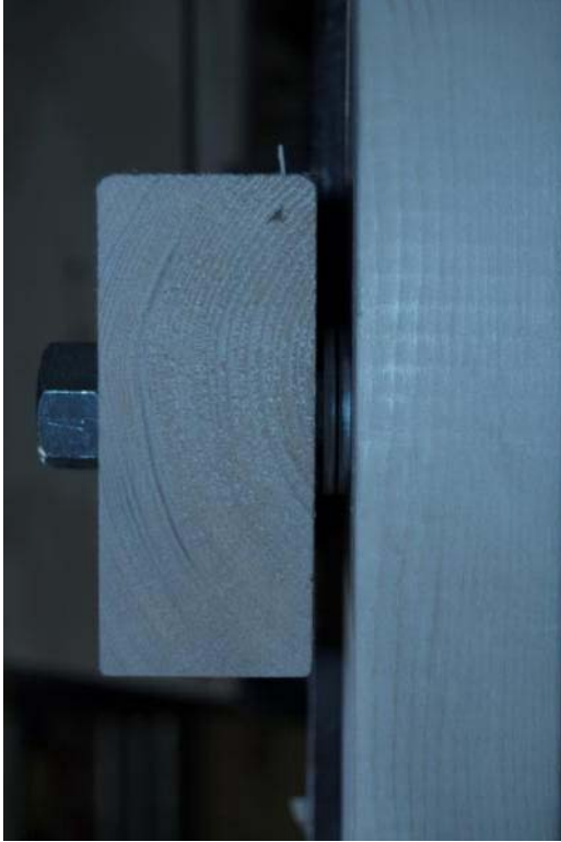
Washers between frame and axle
