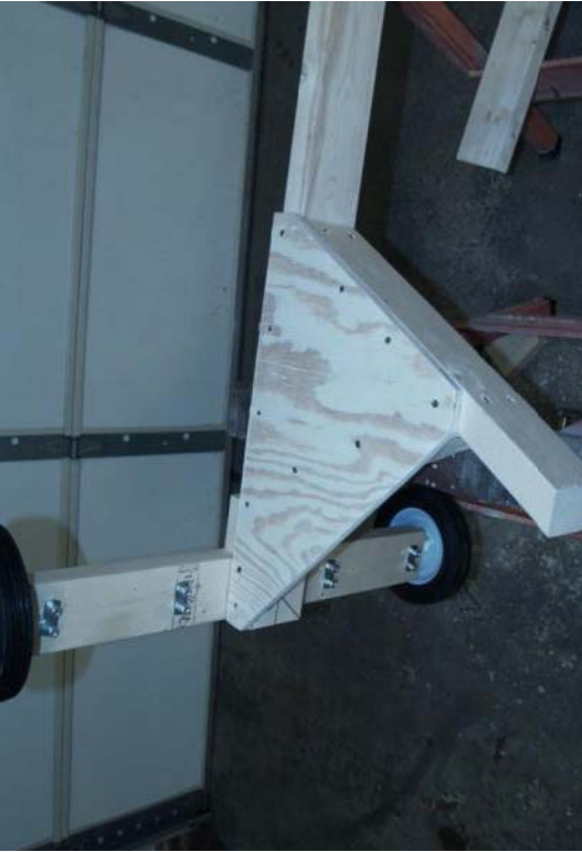
Seat Post and Brace – Side panel installed
