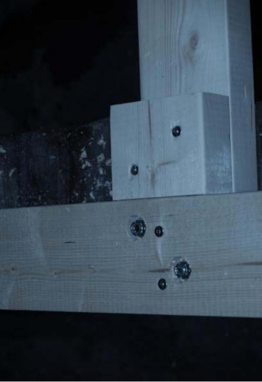
Rear Axle Bottom – Alignment block (optional) enables axle to remain square if it should be removed and re-attached (Transport)
