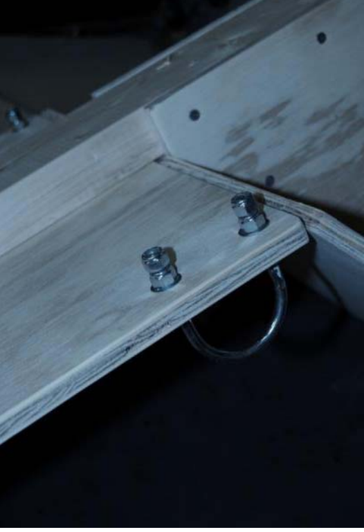
Seatbelt Hardware – Installed, bottom view, double nuts eliminate exposed threads
